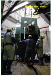
Generator stator being carried into the building [Carry-in completed on October 15, 2012] (Photo taken on October 15, 2012)
