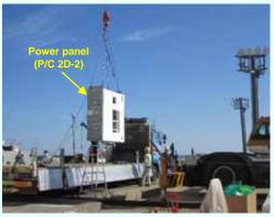
Power panel being lifted up by a crane car (Photo taken on October 16, 2012)
