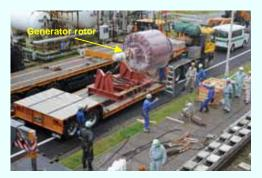
Generator rotor being lifted up by a crane car (Photo taken on October 18, 2012)
