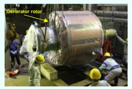
Generator rotor being carried into the building [Carry-in completed on October 18, 2012] (Photo taken on October 18, 2012)
