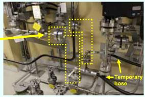
Reactor coolant purification system purge line connected with a temporary hose (Enlarged image) (Photo taken on July 6, 2012)
