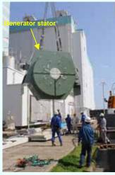
Generator stator being lifted up by a crane car (Photo taken on October 15, 2012)
