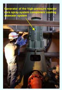
Functional check after the generator installation (Vibration measurement during trial operation) [Permanent installation completed on October 11, 2012] (Photo taken on October 11, 2012)
