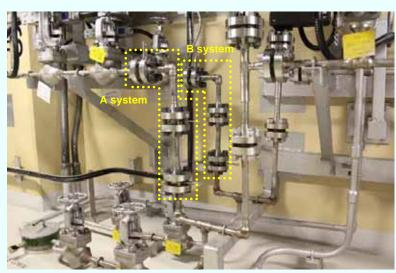
Purge line (A system, B system) after being switched to the permanent pipe [Completed on October 11, 2012] (Photo taken on October 29, 2012)
