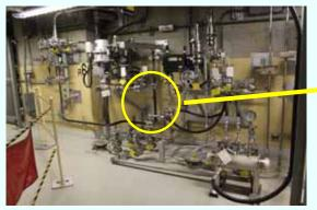
Reactor coolant purification system purge line connected with a temporary hose (Photo taken on July 6, 2012)
