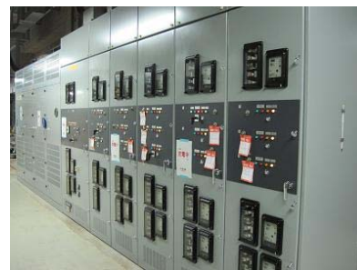
Restored power panel
