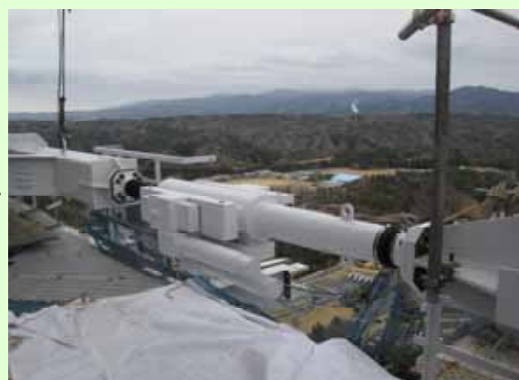
Seismic control oil damper installation completed (Photo taken on April 20, 2012)
