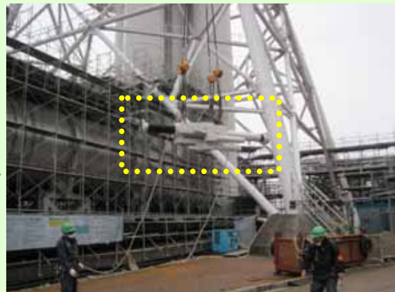
Seismic control oil damper being lifted up (Photo taken on April 20, 2012)
