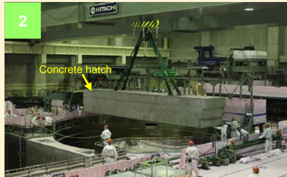
Concrete hatch removal (Photo taken on September 10, 2012)
