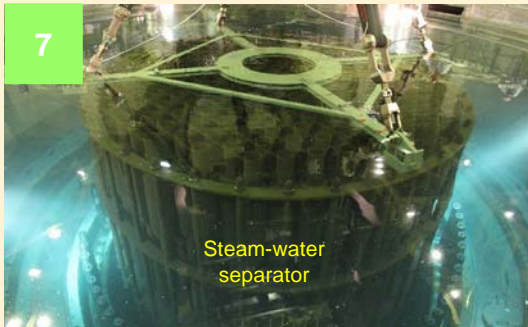
Steam-water separator removal (Photo taken on September 21, 2012)
