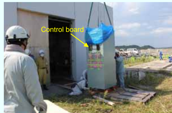
Carry-in of the control board (Photo taken on September 4, 2012)
