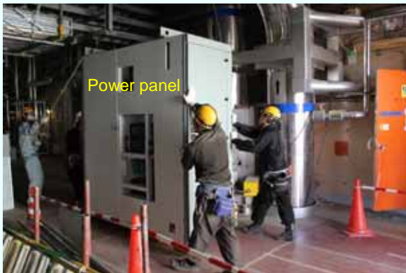
2. Carry-in of the power panel (Photo taken on September 3, 2012)
