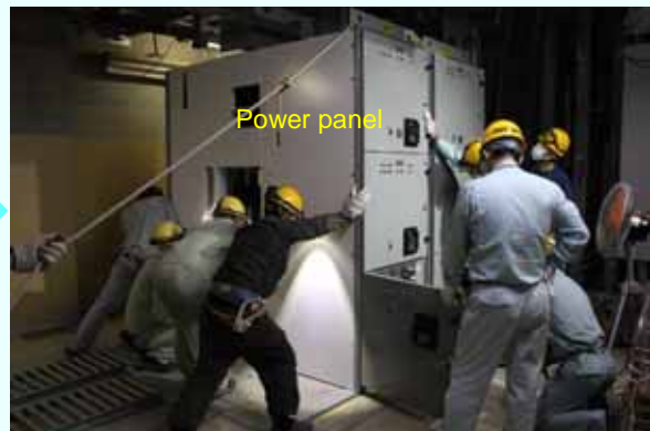
3. Power panel installation (Photo taken on September 3, 2012)
