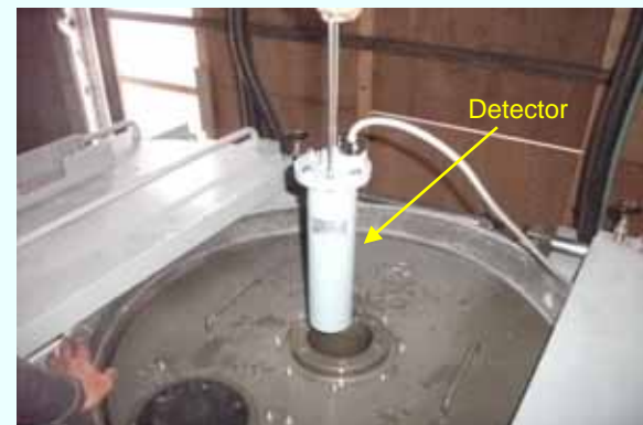
Discharge monitor (detector) installation (Photo taken on September 4, 2012)
