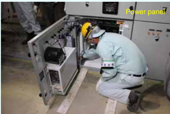
4. Power panel being fixed (Bolt installation) (Photo taken on September 3, 2012)
