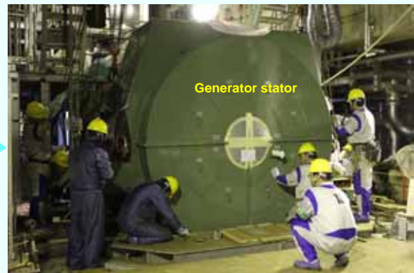
4. Generator stator being installed (Photo taken on August 8, 2012)
