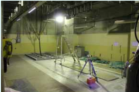
Before installation (Photo taken on June 8, 2012)
