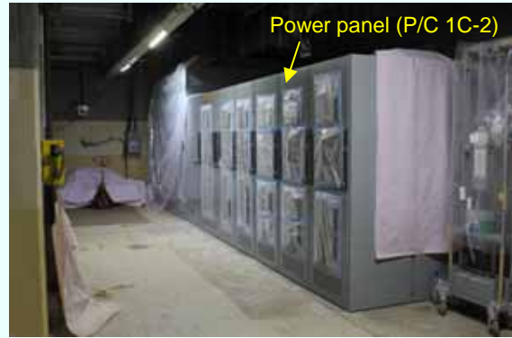
Installation completed on July 10, 2012 (Photo taken on July 24, 2012)
