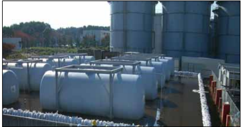
(2) Appearance of outdoor hazardous material storage tank at the “Wild Bird Forest”
