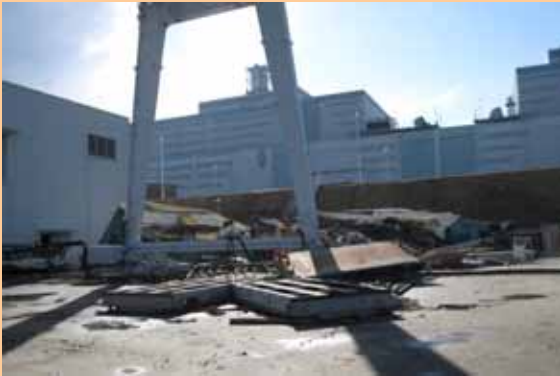
Between Unit 3-4 Seawater Heat Exchanger Buildings (Outside) (Photo taken on March 16, 2011)
