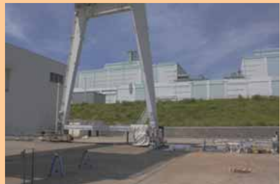
Between Unit 3-4 Seawater Heat Exchanger Buildings (Outside) Debris removal completed (Photo taken on June 21, 2012)
