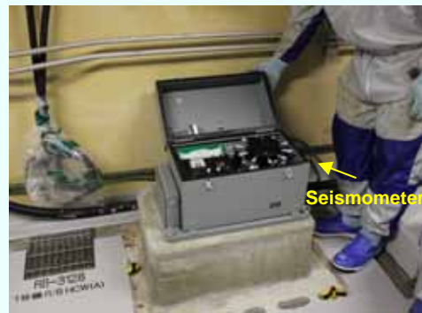
Seismometer installation (Unit 1 Reactor Building 2nd floor) (Photo taken on June 5, 2012)
