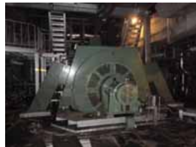
Water damaged Unit 1 D/G (A)
