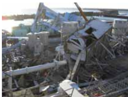
Unit 5 sea side sea water pump area
