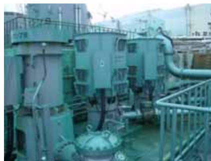
Unit 1 Containment Cooling Spray Seawater System Pump
