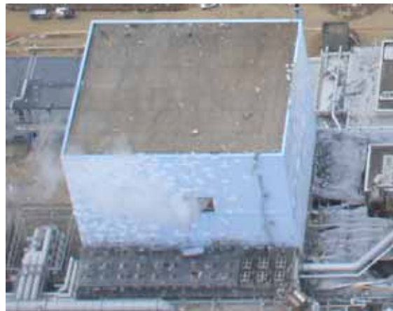
Opening of the Unit 2 blowout panel
