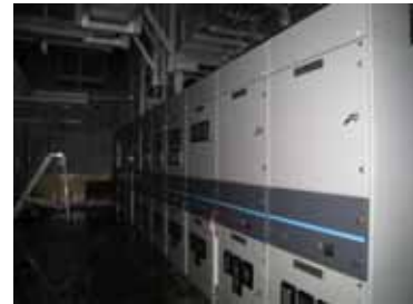
Water damaged Unit 1 M/C power panel (water on floor)
