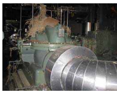
Water damaged Unit 1 RHR seawater system intermediate loop recirculation pump
