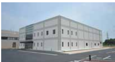
Exterior of the seismic isolated building
