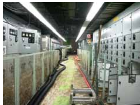
Water damaged Unit 1 T/B 1F P/C
