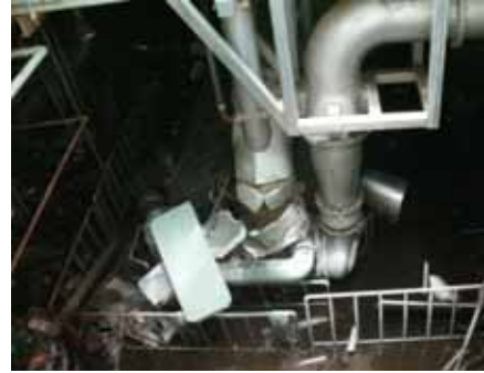
Water damaged Unit 1 D/G (1B)
