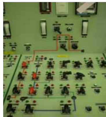
HPCI control panel (photo taken at later date) At the time, all condition indicator lamp were off
