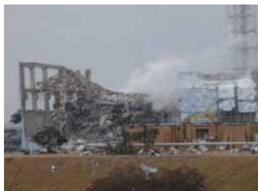
Unit 4 damage (on right side of photo) (Unit 2 is on left side of photo)
