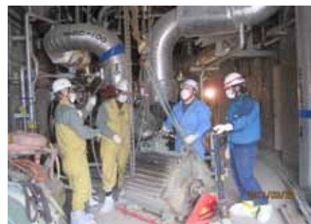
Pump motor restoration work (work conditions shown took place on later date)
