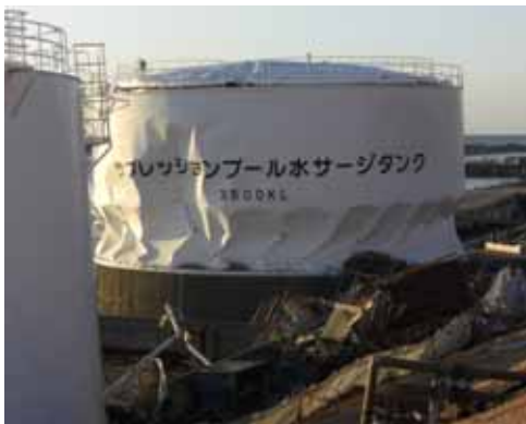
Tank deformed by the tsunami (Same tank shown in picture above)
