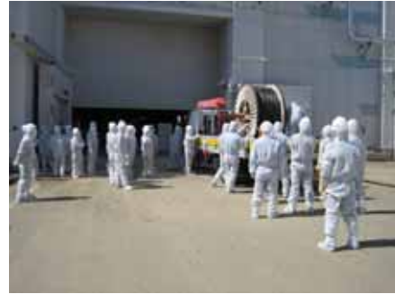
Temporary cable installation preparations (work conditions shown took place on later date)
