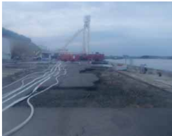
Injection via fire engines at unloading wharf
