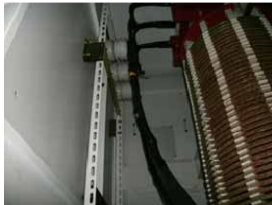
Cable connections to power panel. The 3 wire cable terminals are affixed with bolts and then wrapped with insulation tape.
