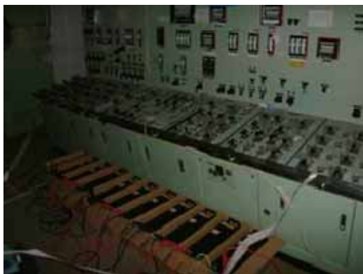
Temporary batteries were connected to instruments to power them
