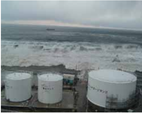
Tsunami destroys 10m high seawall and pushes inland
