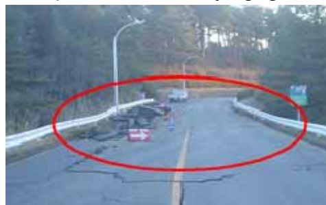
Damage to the access road to Unit 5, 6 (After restoration, the asphalt on one side was stripped off and gravel and rocks underneath were used to restore the other side.)
