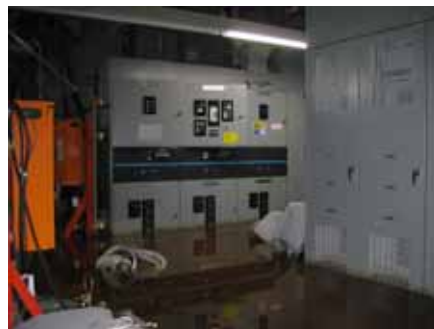
Unit 6 electric item room flooding status
