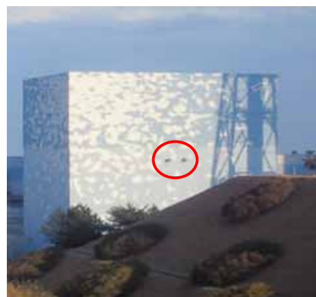
IC vent pipe (nicknamed “pig’s nose”)
