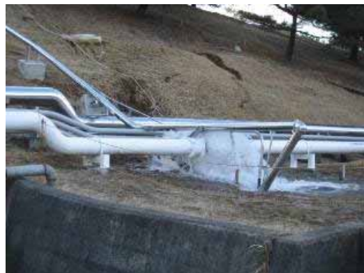
Transformer FP pipe leakage
