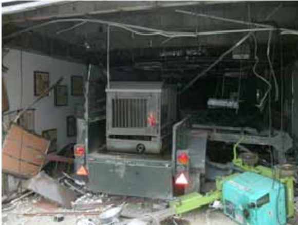
Low voltage. Needed to be towed since the generator was loaded on a trailer (photographed in the days after the disaster)
