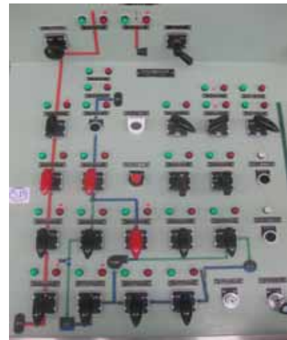
RCIC control panel (taken at a later date)
