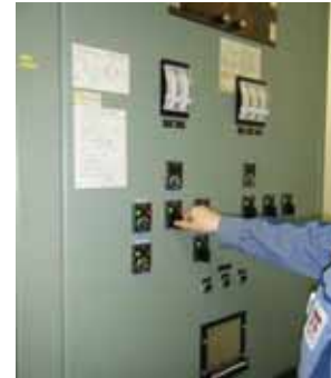
Valve operation with the MCR AM panels (work conditions shown took place on later date)
