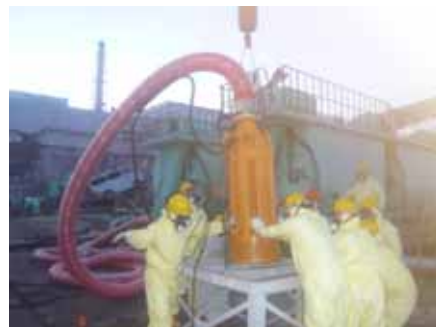
Underwater pump installation work
