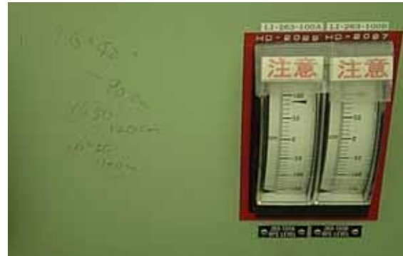
Reactor water level readings temporarily confirmed (read values written next to gauge, monitoring continued)
