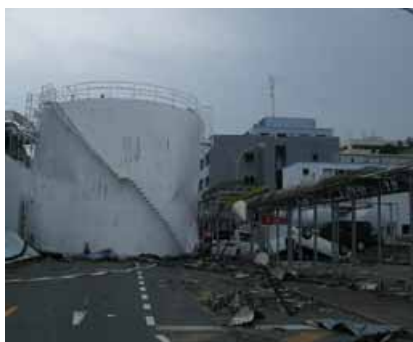
Heavy fuel oil tank swept up by the tsunami and blocking the road (Diameter: 11.7m Height: 9.2m)
