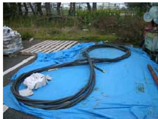
The cable in the photograph is approximately 15m long and weighs approximately 90kg. A cable more than 10 times this length was used to restore power to Unit 1 and 2 (photographed in the days after the disaster)
