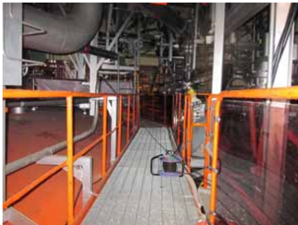
Torus room conditions (Unit 5, with light)
