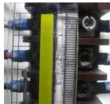
Terminal block (photo taken at later date) Wires were connected to a terminal block approx. 1cm wide
