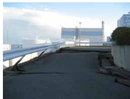
Site road cracked and impassable
