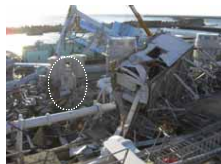
Seawater pump area status
