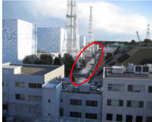
Units 1 to 4 flooded by tsunami
