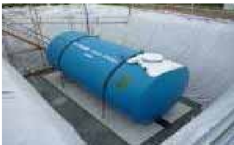
Buried FP tank (taken at time of installation)
