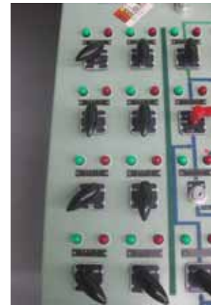
SRV control panel (taken at a later date)
