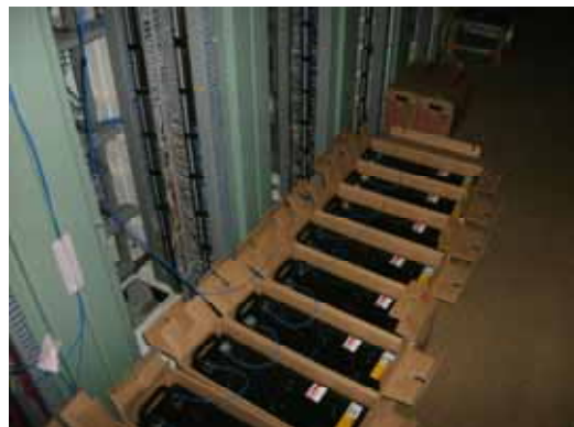
Ten 12V battery parallel[in series] (photo taken at a later date, with light)
