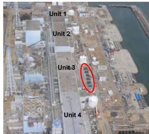
Unit 3 backwash valve pit
