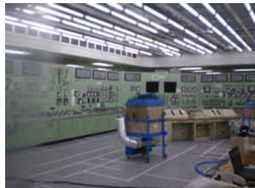
Unit 1 and 2 Main Control Room (photo taken afterwards)
