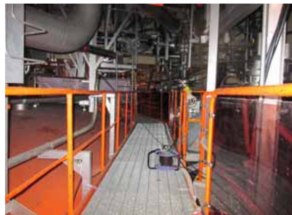
Catwalk (Unit 5, with light)
