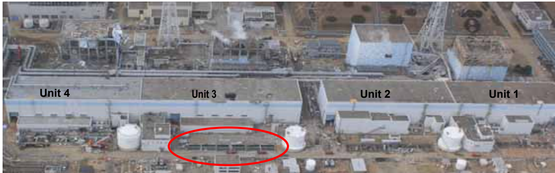
Unit 3 backwash valve pit
