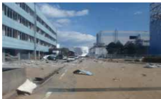
Former main office, where windows were broken by blast winds (Unit 1 can be seen to the right)
