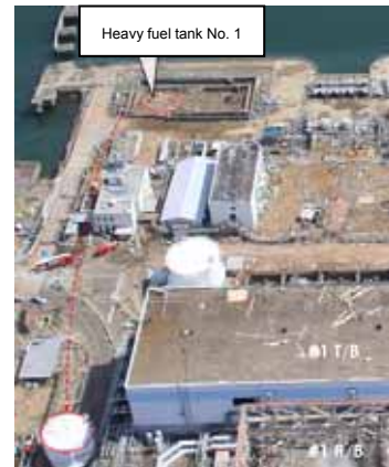
The heavy fuel tank was carried to the north side of the Turbine Building by the Tsunami
