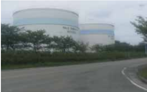
Filtered water tank
