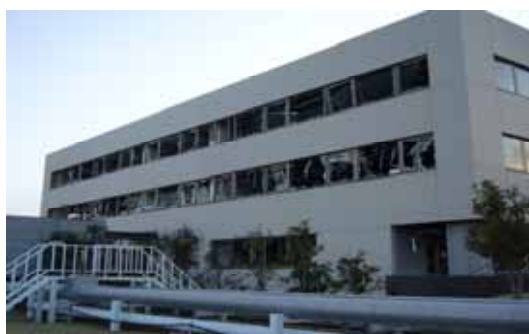
Main office, where windows were broken by blast winds
