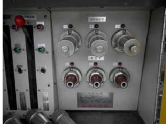
Tohoku Electric high voltage. As with high-voltage, temporary cables needed to be laid and terminals processed in order to send power to the P/C (photographed in the days after the disaster)
