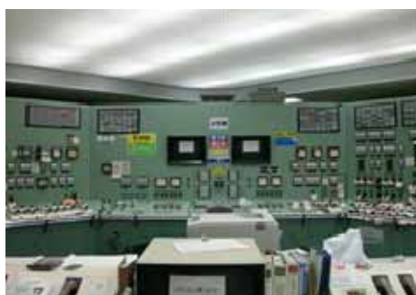
MCR light restoration (Unit 4)
