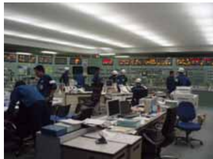
Units 5 and 6: Unit 6 side
