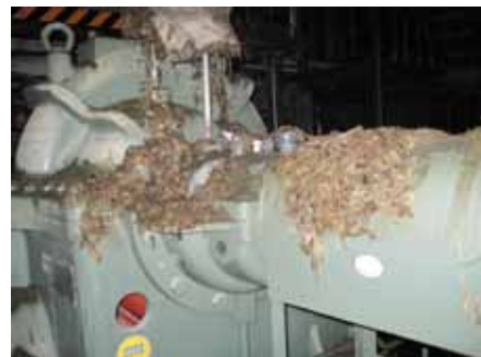
Water damaged cooling water pump (photo taken at later date)
