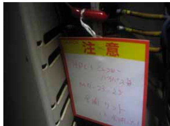
HPCI control panel
