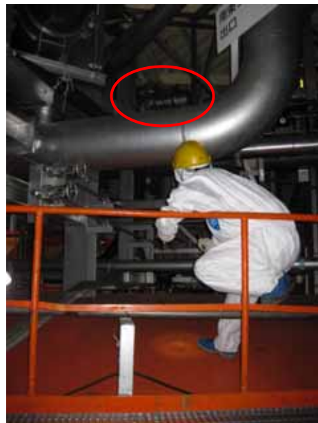
S/C vent valve check (example)
