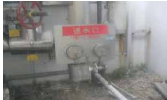
Unit 1 FP line intake
