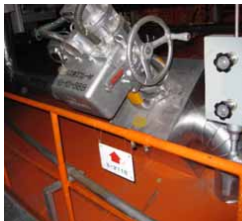
S/C spray valve (Unit 5 side, with light)
