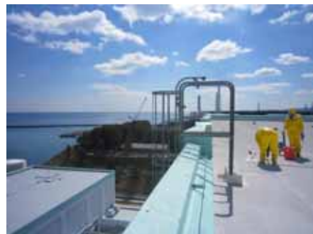
Work on the rooftop
