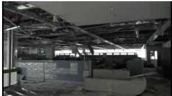
State of the Main Office
