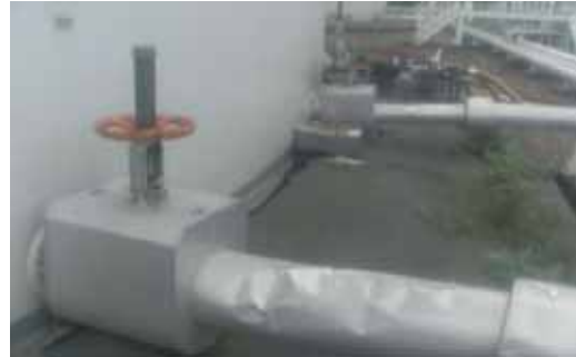
Tank outlet valve near filtered water tank
