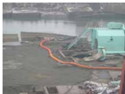
Underwater pump installation status (installation took place on later date)
