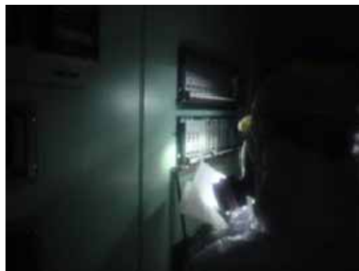
Indicators were checked using flashlights
