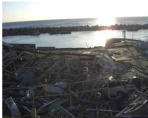
Conditions on sea side after tsunami arrival
