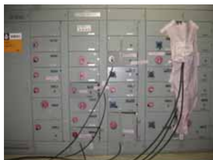
Temporary power source cable connection status (photo taken at later date)
