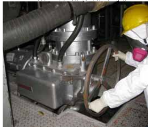
Example of RHR injection valve operation (Unit 5, with light)
