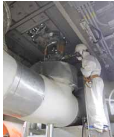
RHR injection valve installed on piping approx. 60cm in diameter (Unit 5, with light)
