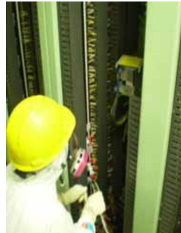
Behind the control panel (photo taken at a later date, with light)
