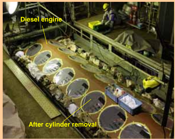
Recovery work for Unit 1 D/G (H) (Photo taken on April 17, 2012)
