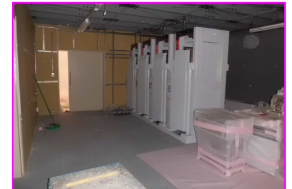
⑥ Installment of gate monitors
