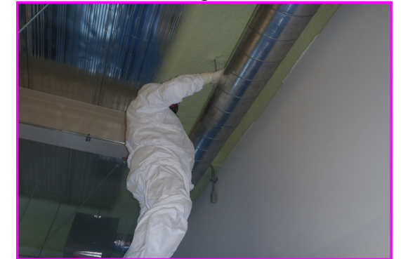
④ Removal of ducts
