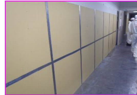
① Sticking lead boards to inside walls
