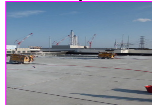
⑤ Removal of roof concrete
