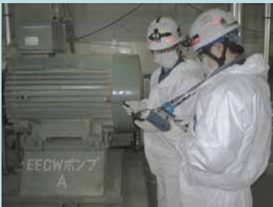
Vibration diagnosis (Photo on March 28, 2012)
