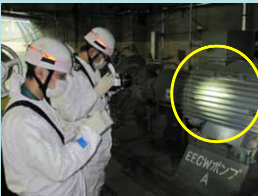
Infrared thermography diagnosis (Photo on March 28, 2012)
