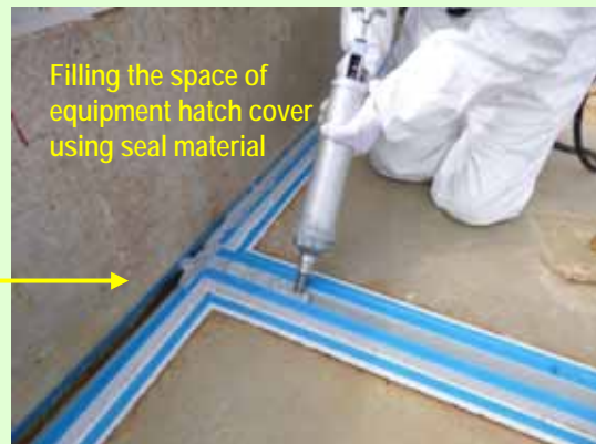
Filling the cover space using seal material (Photo on March 23, 2012)
