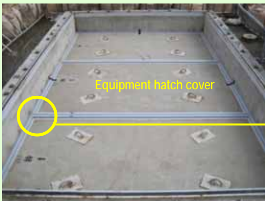
Watertight of the cover space using seal material (Photo on March 23, 2012)
