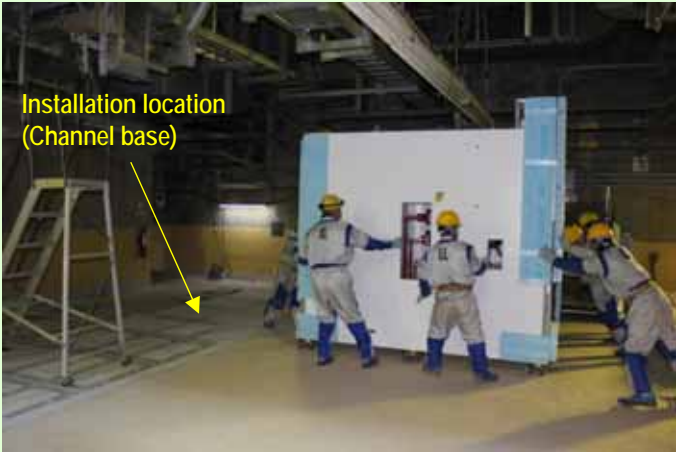
(3) Moving after lift down (Photo on March 15, 2012)
