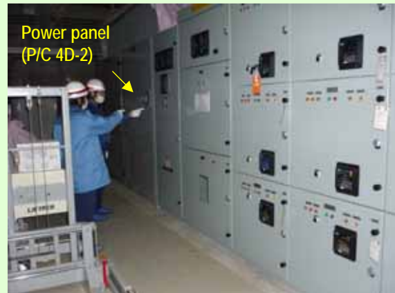
Function check (Function check and switch to permanent installation was completed on March 23, 2012) (Photo on March 23, 2012)
