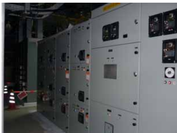
Power panel (permanent installation) (Recovered on January 30, 2012) (Photo on February 24, 2012)
