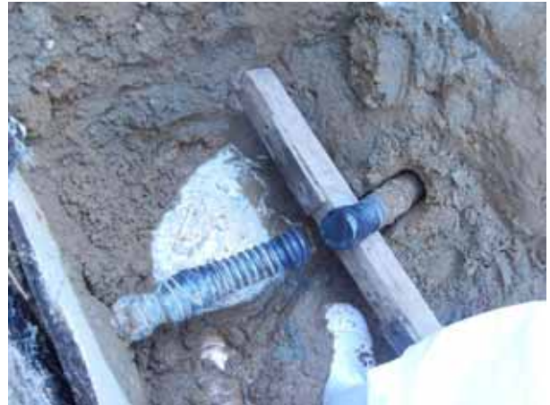
Figure4 Before and after the cutting of cable conduit line
