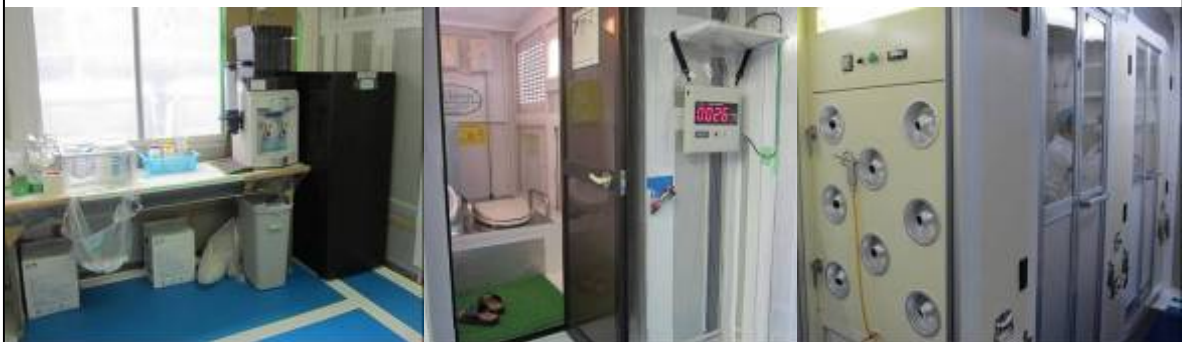
Inside of on-site rest stations (from left: drinking water, etc., restroom and air shower)
