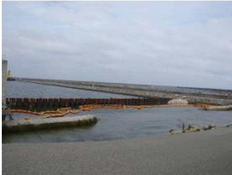
Status of steel pipe sheet pile
