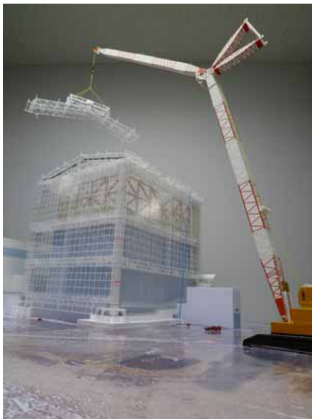
Photo 2 Model used for examining installation of cover for the reactor building of Unit 1
