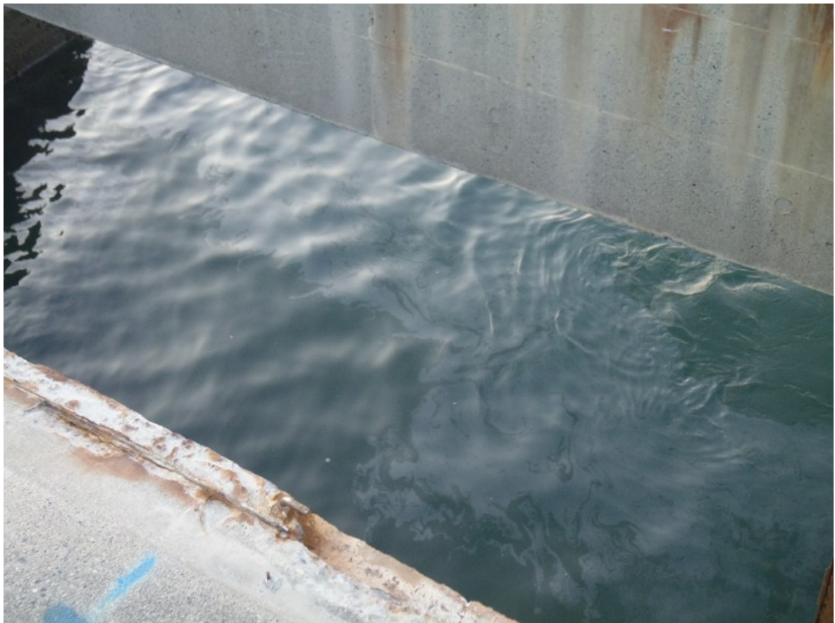
Oil leakage found around water discharge canal of Unit 3, 4
