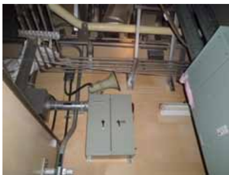
internal wall, 1FL
