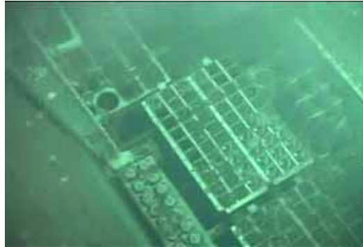
Figure 3: the status inside the spent fuel pool (taken on April 28)
