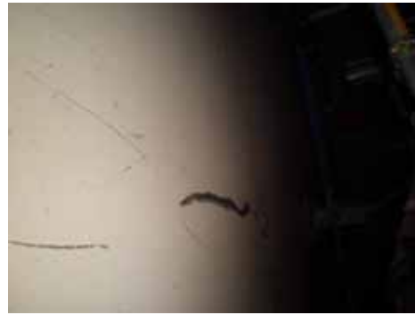
external wall, 2FL
