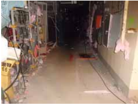
Floor on the second floor
