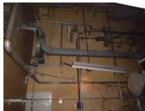
external wall, 1FL
