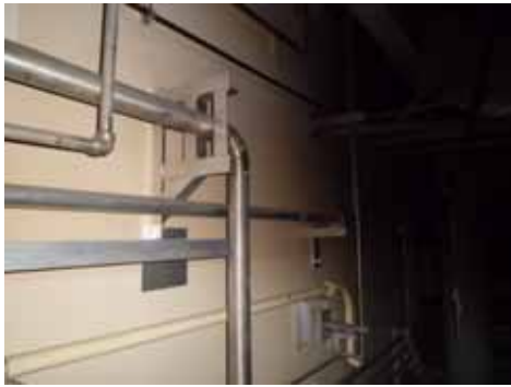
internal wall, 2FL
