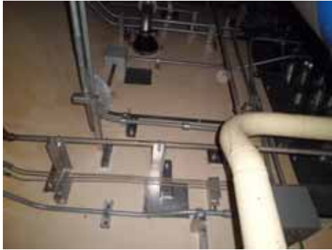
Exterior Wall on the first floor
