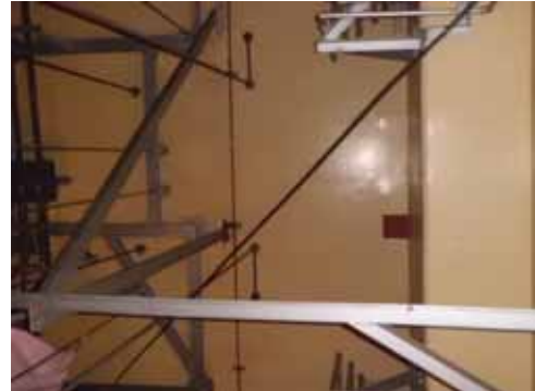
Lower Part of Spent Fuel Pool
