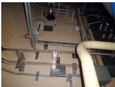
external wall, 1FL
