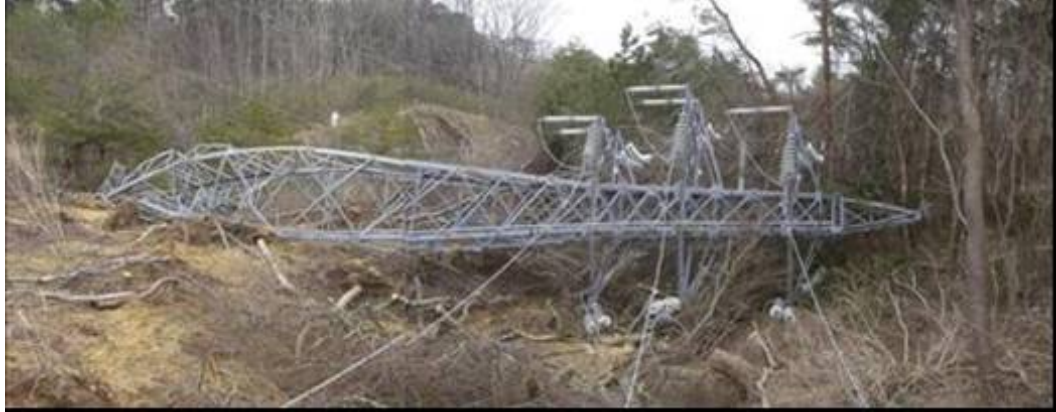
Figure 2: the overall transmission line tower
