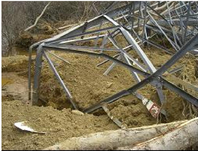
Figure 3: legs of transmission line tower
