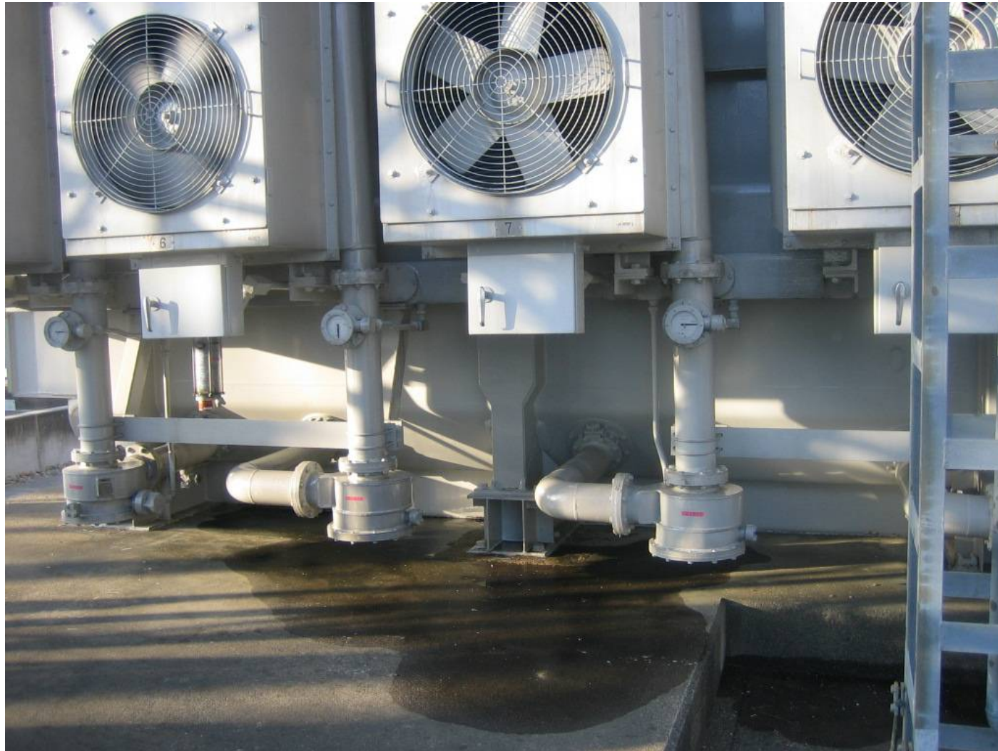
Photo : Tokyo Electric Power Company, March 12, 2011
