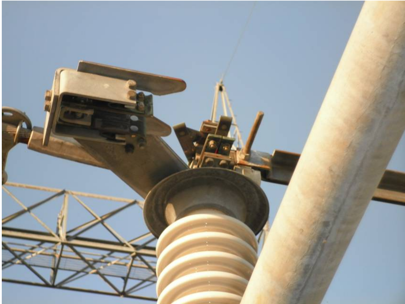
Photo : Tokyo Electric Power Company, March 12, 2011
