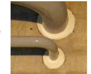
Waterproofing Building Hole
