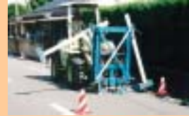
Vibration-generating truck C (with a board pounder) (exploration depth: approx. 30m)
