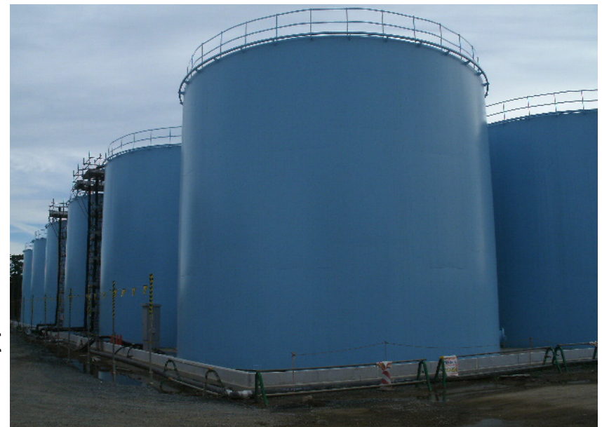
Steel Cylindrical Tank (Welded-Type)
