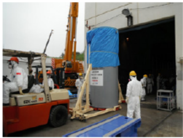
Installation of Cesium Adsorption Vessel
