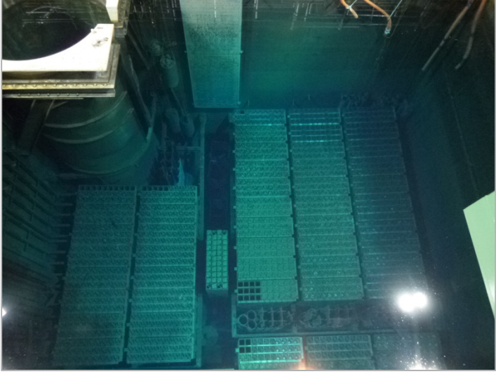
SFP after the removal of felled debris Photographed on November 5, 2013
