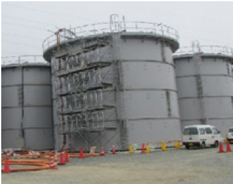
Steel Cylindrical Tank (Flange-Type)
