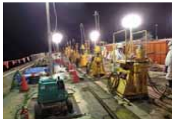
<Ground improvement construction>
