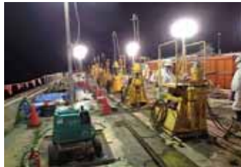
<Ground improvement construction>
