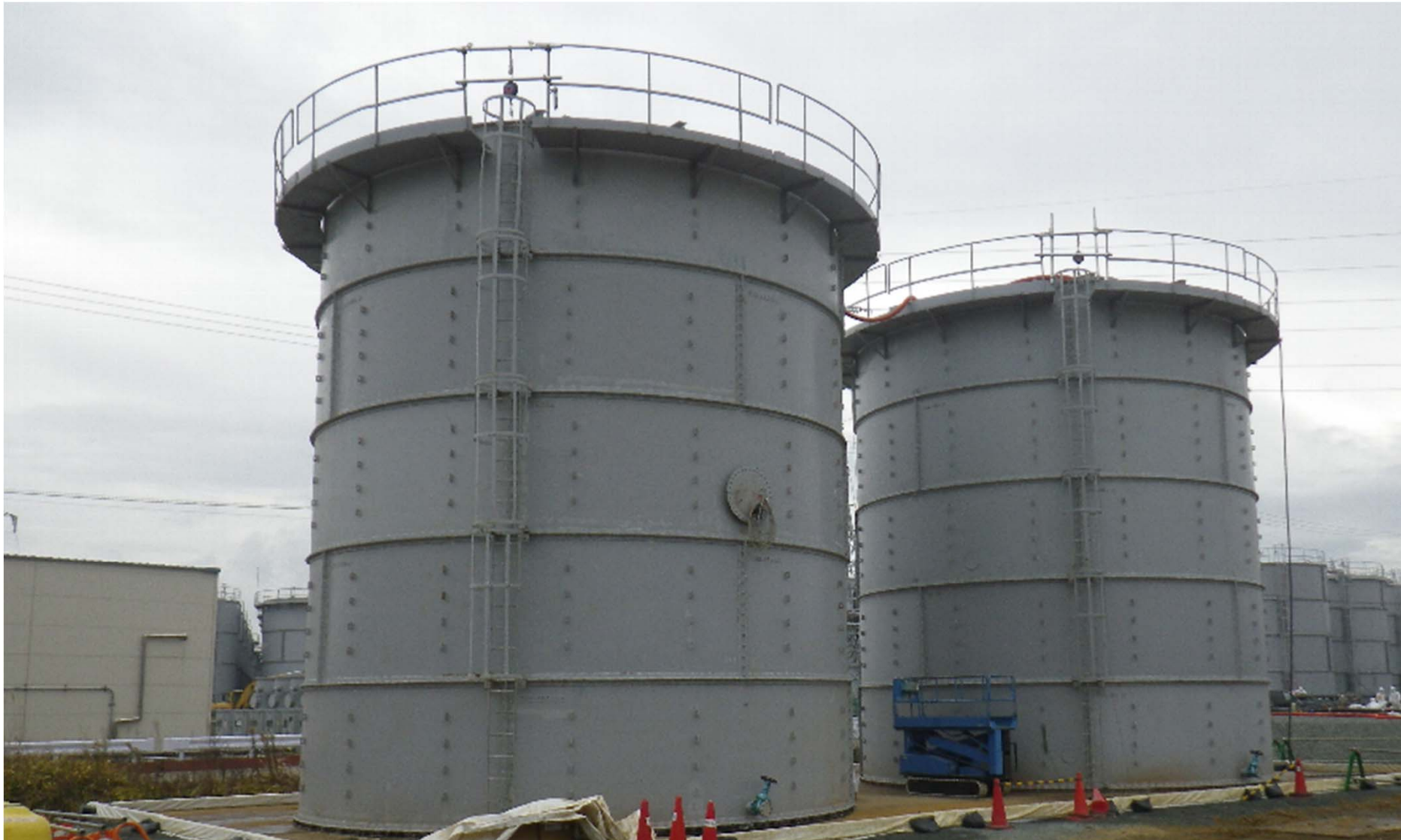
New tanks installed
