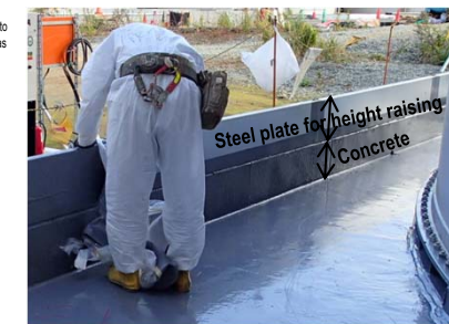
Status of height raising of fences by steel plate
