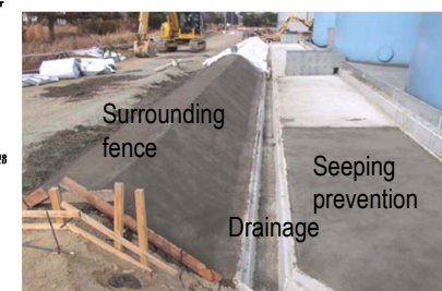
Status of facing over ground surface around tanks
