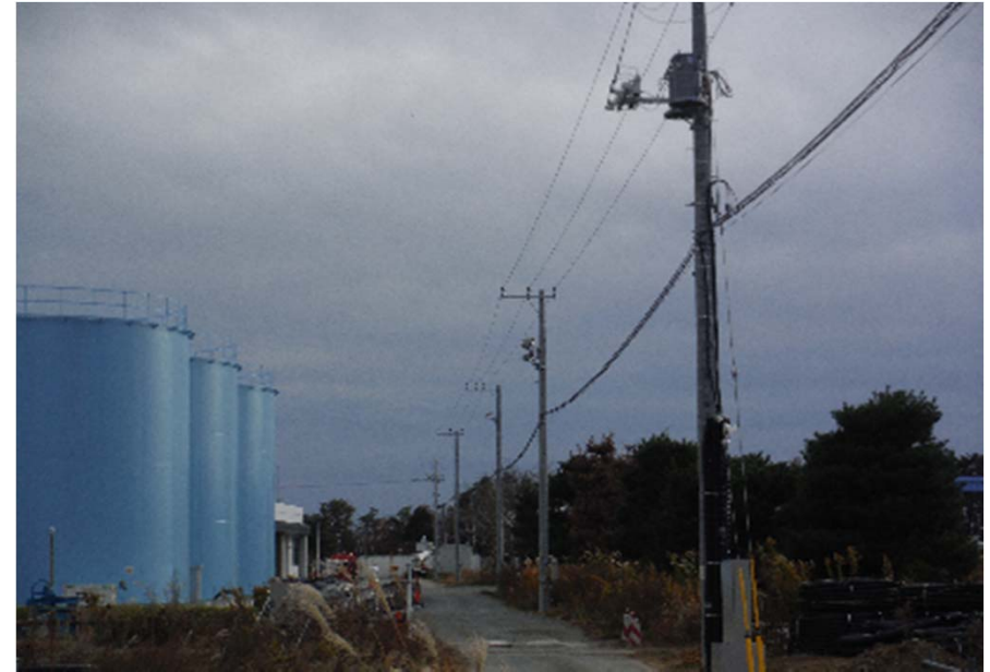
Zone E installation status of distribution lines and lighting facilities
