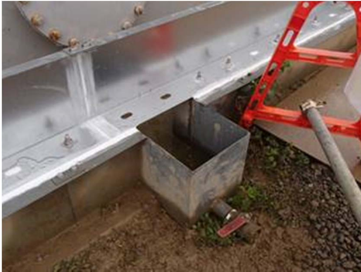
Catch basin before closure (outside)
