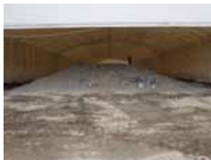
Debris transportation completed (in the first storage facility) (November 19)
