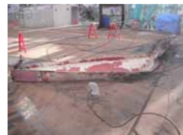
Steel beam after being removed
