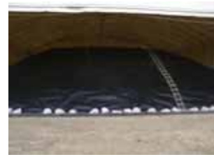
Impermeable liner installation in progress (in the first storage facility) (December 13)
