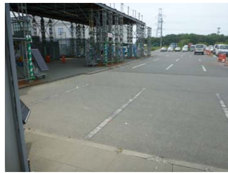
Before iron plate installation
