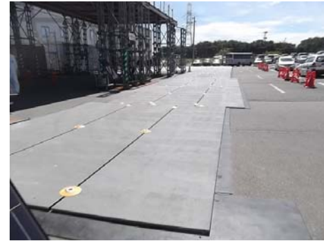
After iron plate installation
