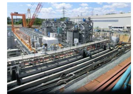
2. Multi-nuclide removal equipment installation (August 19)
