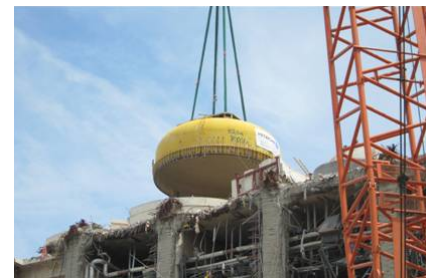
Lifting down PCV upper lid
