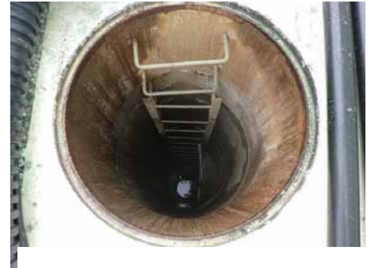
Inside of the Sub-drain pit
