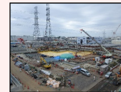
After dismantling in H1 east area
