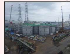
Start of dismantling in H1 east area
