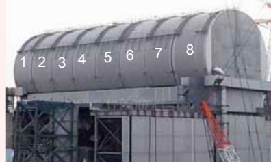
Installation of dome roof (February 21)
