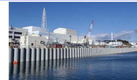
(Sea-side impermeable wall)
