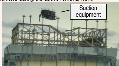
<Installation status (January 22)>
