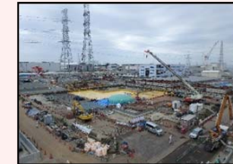
After dismantling in H1 east area
