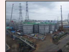
Start of dismantling in H1 east area
