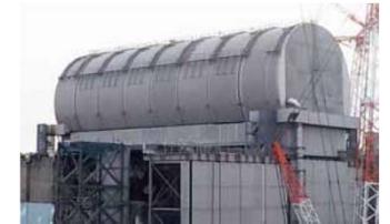
Installation of dome roofs (February 21, 2018)
