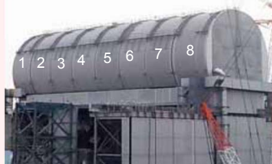
Installation of dome roof (February 21)
