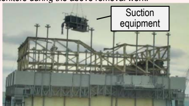
<Installation status (January 22)>
