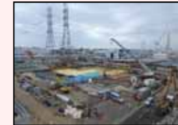
After dismantling in H1 east area
