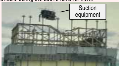
<Installation status (January 22)>
