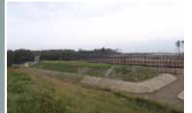
Temporary soil-covered type storage facility
