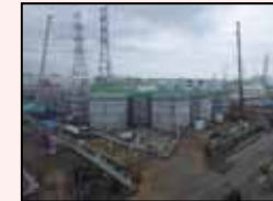
Start of dismantling in H1 east area
