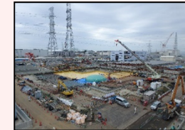
After dismantling in H1 east area
