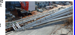
(Installation of brine pipes)
