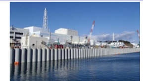
(Sea-side impermeable wall)
