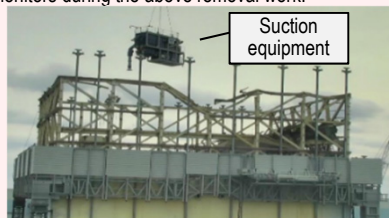
<Installation status (January 22)>
