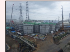
Start of dismantling in H1 east area
