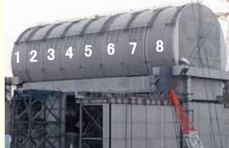
Installation of dome roofs (February 21, 2018)
