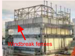
<Installation status (December 19)>
