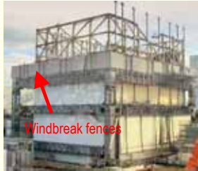
Installation status (December 19)
