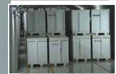
Solid waste storage facility
