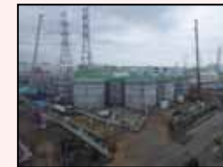
Start of dismantling in H1 east area
