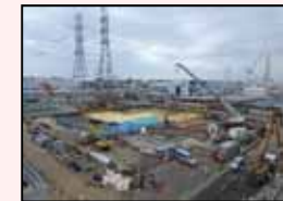
After dismantling in H1 east area
