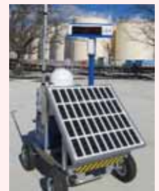
Installation of Dose-rate monitor
