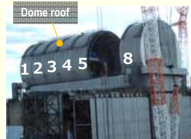
Installation of the fuel removal cover (December 19, 2017)
