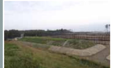
Temporary soil-covered type storage facility
