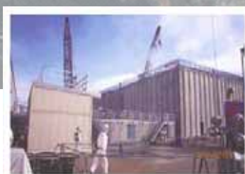
Temporary waste sludge storage
