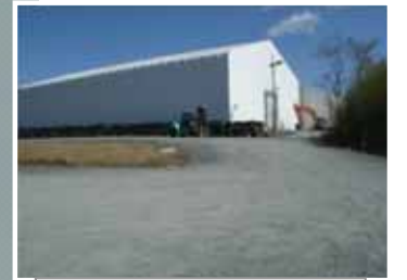
Rubble storage tent
