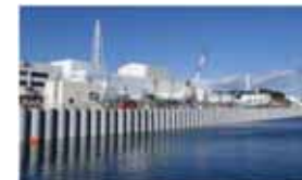
(Sea-side impermeable wall)
