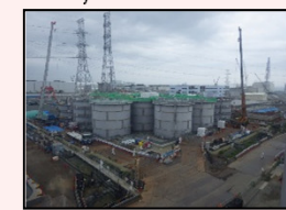
Start of dismantling in H1 east area
