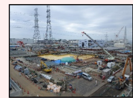
After dismantling in H1 east area
