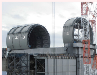
Installation of dome roof (October 25)
