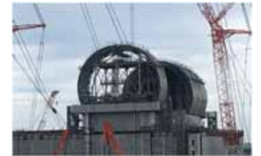
Installation of a cover for fuel removal at Unit 3 (October 25, 2017)
