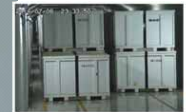
Solid waste storage facility
