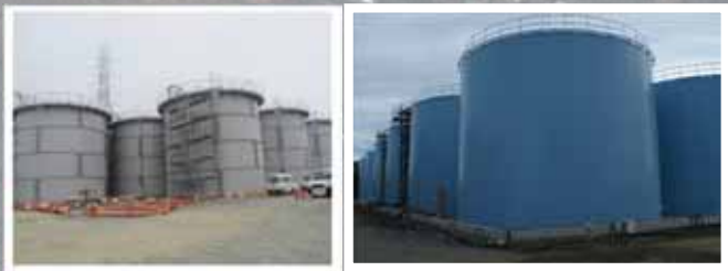
Tank installation status
