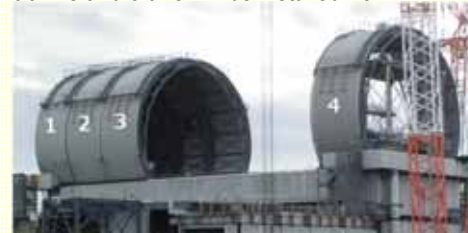
<Installation of dome roof (October 25)>
