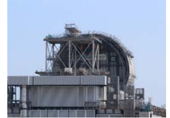
Installation of a cover for fuel removal at Unit 3 (September 27, 2017)
