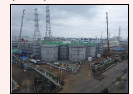
Start of dismantling in H1 east area
