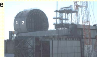
<Installation of dome roof (September 26)>
