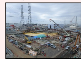
After dismantling in H1 east area
