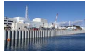
(Sea-side impermeable wall)
