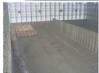
Inside the rubble storage tent
