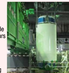
Fuel removal status
