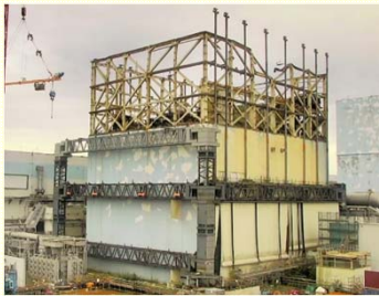
Unit 1 building cover <Installation of north-side pillars and beams> (photo from the northwest side on August 31)
