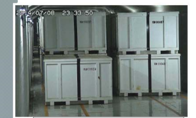
Solid waste storage facility
