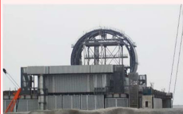
Installation of a cover for fuel removal (photo taken on August 5, 2017)
