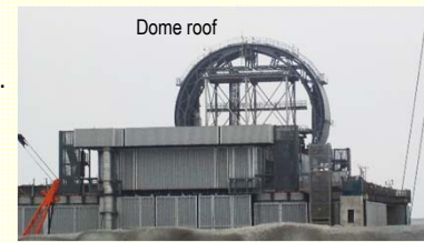
<Installation of dome roof (Photo on August 5)>
