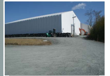
Rubble storage tent
