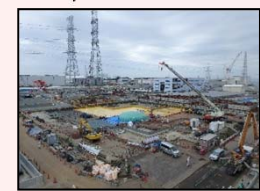
After dismantling in H1 east area
