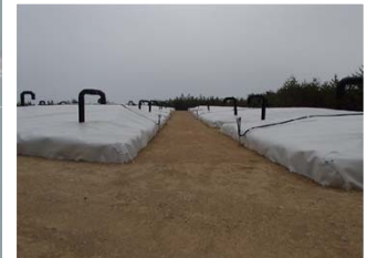
Temporary trimmed trees storage pool
