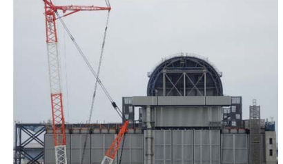
Installation of a cover for fuel removal at Unit 3 (August 28, 2017)
