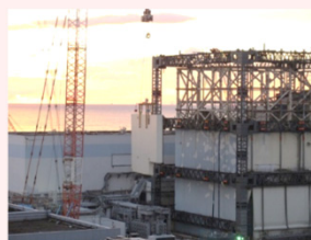
<Dismantling of wall panels>
