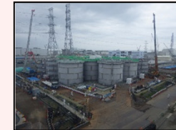
Start of dismantling in H1 east area
