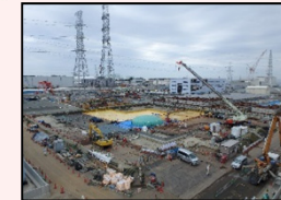
After dismantling in H1 east area
