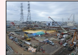
After dismantling in H1 east area
