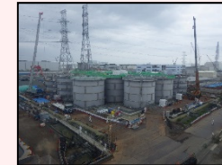
Start of dismantling in H1 east area
