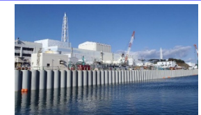
(Sea-side impermeable wall)
