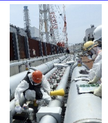
(Opening/closure of frozen pipes)
