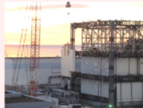
<Dismantling of wall panels>
