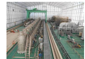
(High-performance multi-nuclide removal equipment)
