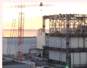
<Dismantling of wall panels>
