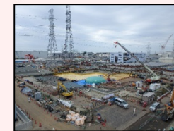
After dismantling in H1 east area
