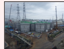
Start of dismantling in H1 east area
