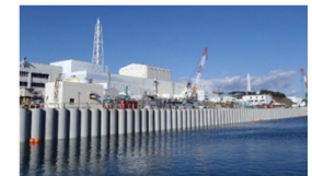
(Sea-side impermeable wall)
