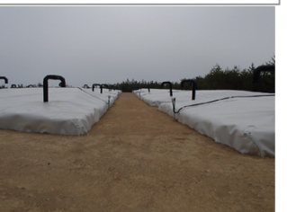
Temporary trimmed trees storage pool
