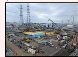
After dismantling in H1 east area
