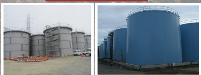
Tank installation status
