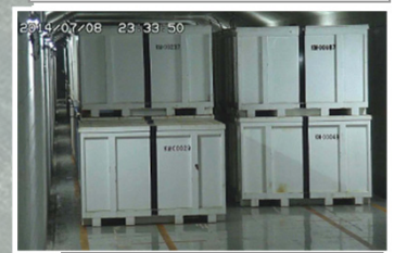
Solid waste storage facility
