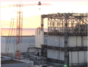
<Dismantling of wall panels>
