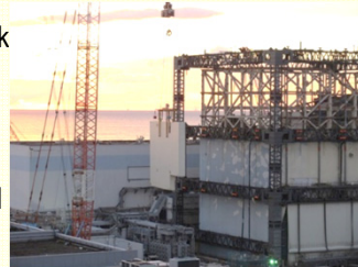
<Dismantling of wall panels>
