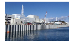
(Sea-side impermeable wall)
