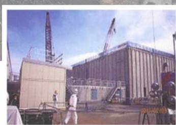
Temporary waste sludge storage
