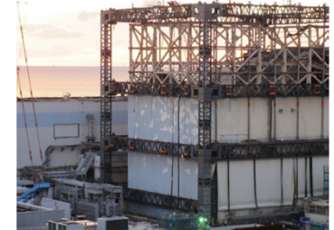
(Dismantling of Unit 1 building cover wall panels)
