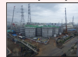
Start of dismantling in H1 east area
