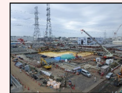
After dismantling in H1 east area
