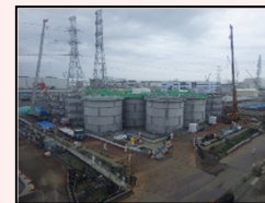
Start of dismantling in H1 east area
