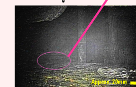
Investigation inside PCV
