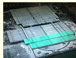
<Installation of shields>
