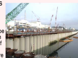
Installation of steel pipe sheet piles for sea-side impermeable wall
