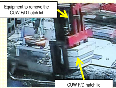
<Removal of CUW F/D hatch lid>
