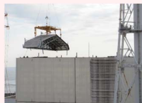
Status of removal of roof panels
