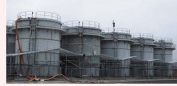
After installing the fence cover
