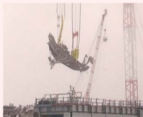
Removal of fuel-handling machine on August 2
