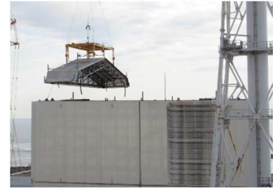
(Dismantling of the Unit 1 building cover)
