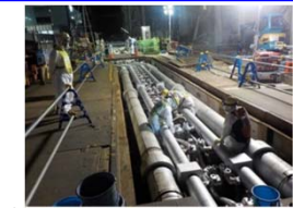
(Installation of pipes for land-side impermeable walls)
