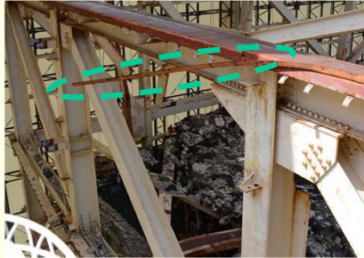
<Example of interfering steel frames to be removed>
