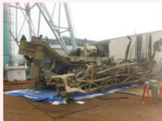
Fuel handling machine removed from the pool
