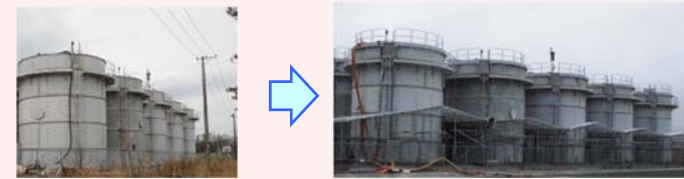
Before installing the fence cover
