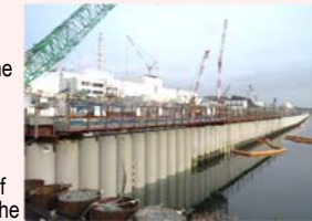
Installation of steel pipe sheet piles for sea-side impermeable wall
