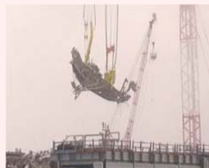
Removal of fuel-handling machine on August 2
