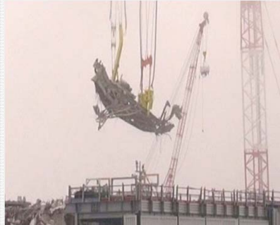
<Removal of the fuel-handling machine>
